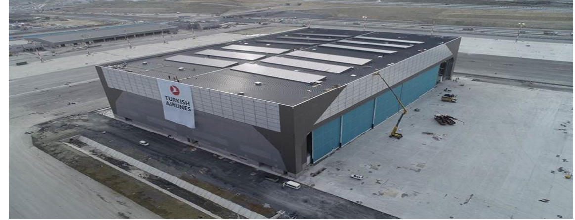
İstanbul Airport THY LMH Building
